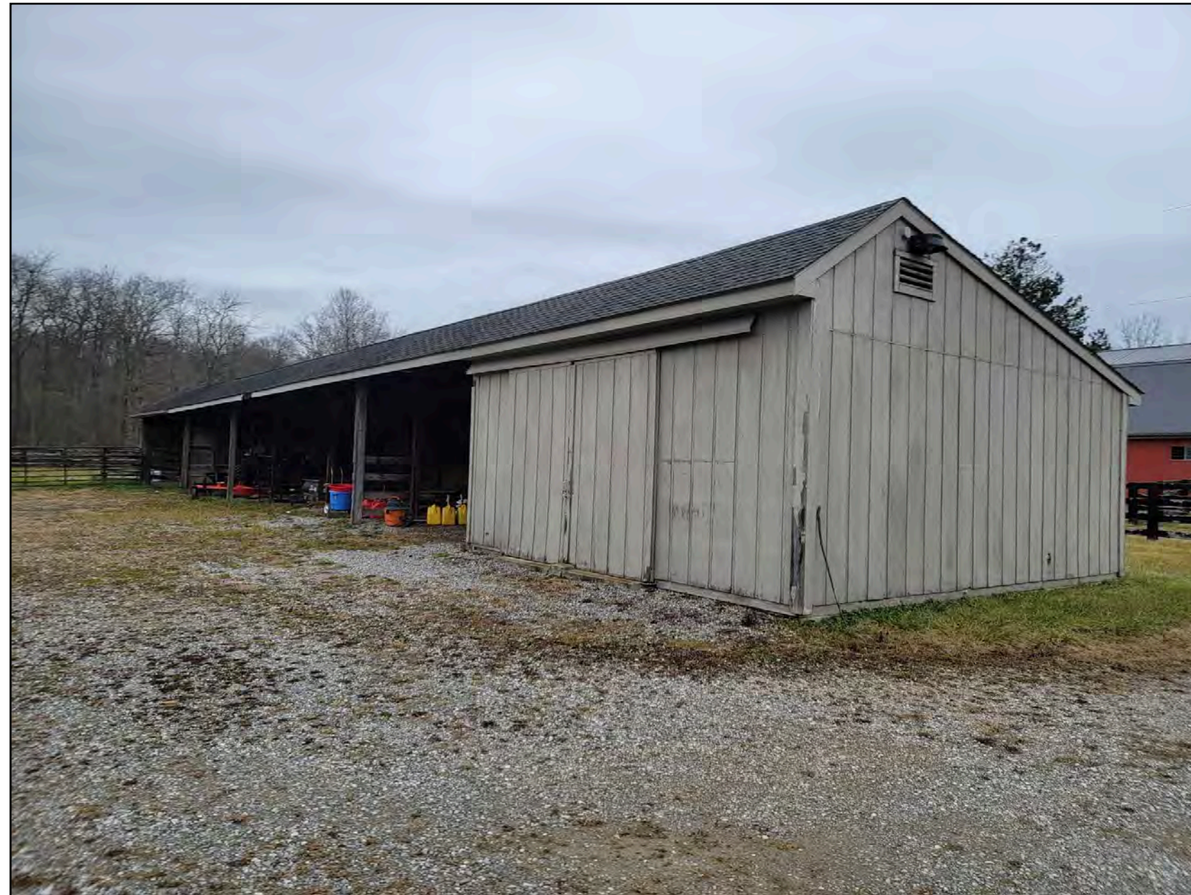
Maintenance Barn "E"
