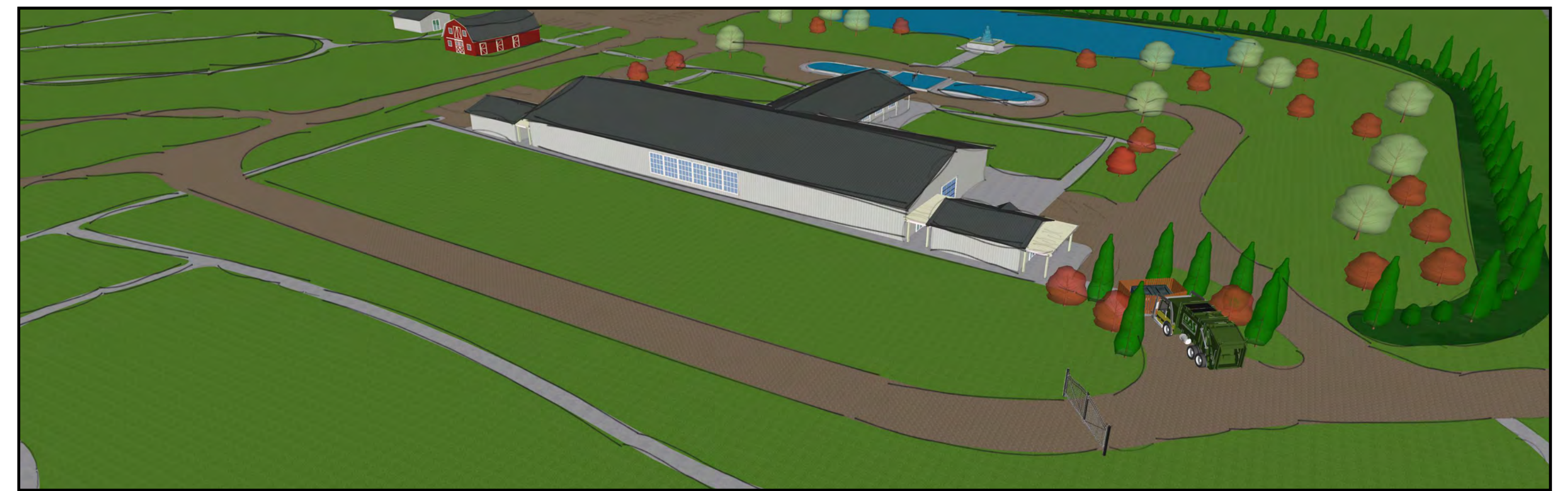
View of Rear of Main Facility
