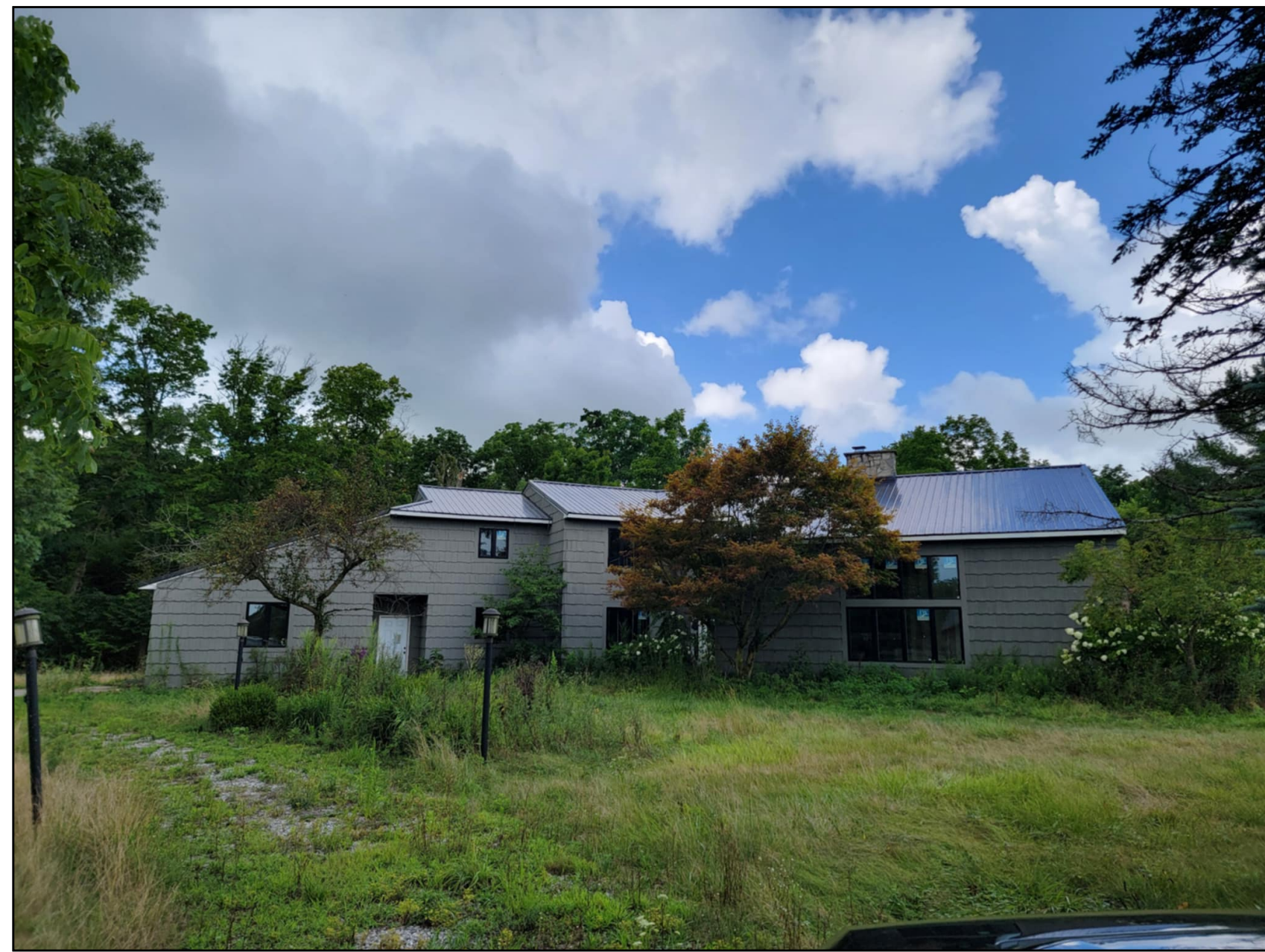
Office / Preparation Building "11" 6112 GABLE ROOF, WOOD SIDING, STEEL ROOFING
