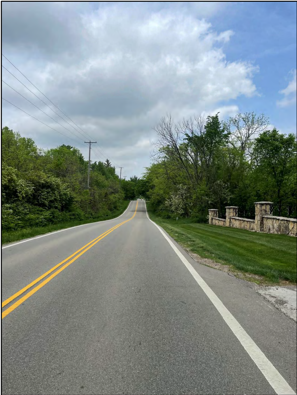
Photo 2 – Sight Distance, 665' North of Proposed Access
